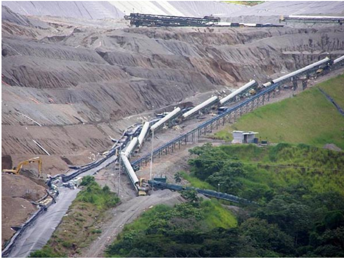
Mining damage in Bellavista, Costa Rica (photo: Scott Cardiff, Earthworks)
