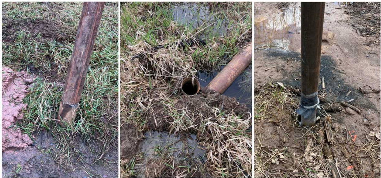
Sealing damage and open pipe photos with discolored ground (Source: DNR 2023-11-08 left, 2024-05-01 center, 2023-05-09 right).
