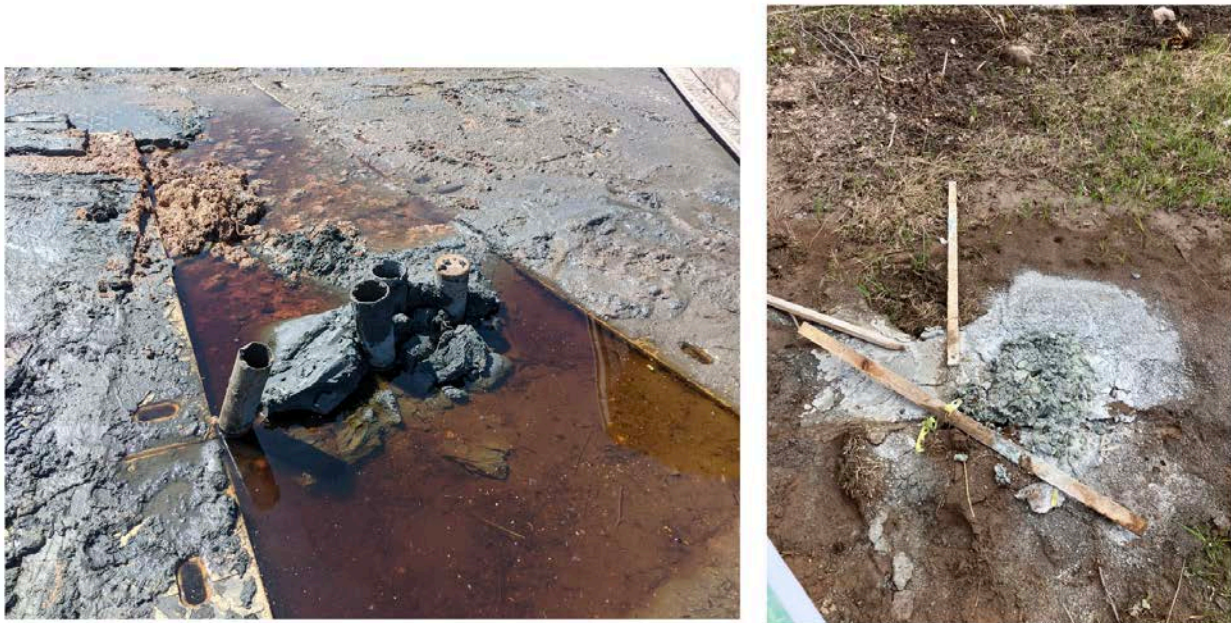
Exposed and buried borings and cracked mats raising pollution concerns (Source: DNR 2022-05-27 left, 2023-05-09 right).
