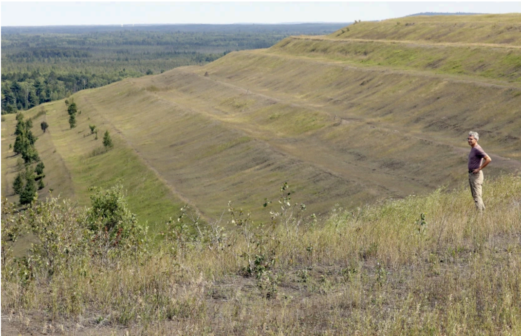
Brad Moore, then PolyMet's executive vice president of environmental and governmental affairs, looks out from the top of a tailings basin dam built when LTV mined taconite near Hoyt Lakes in 2017. Steve Kuchera / File / Duluth Media Group
