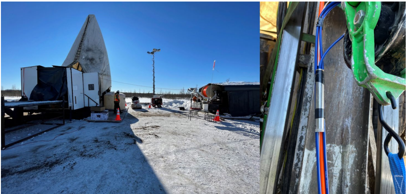
Figure 20.6: Talon Installing Vibrating Wire Piezometers in Exploration Boreholes
