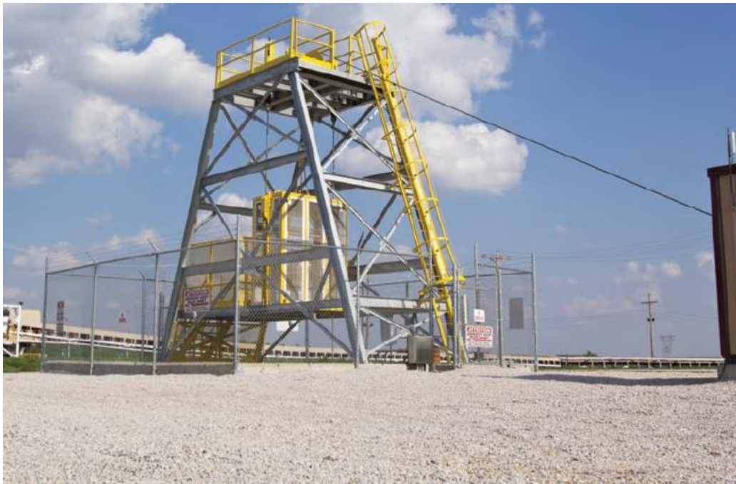
Figure 16-18: 4-Person Emergency Egress Hoist
