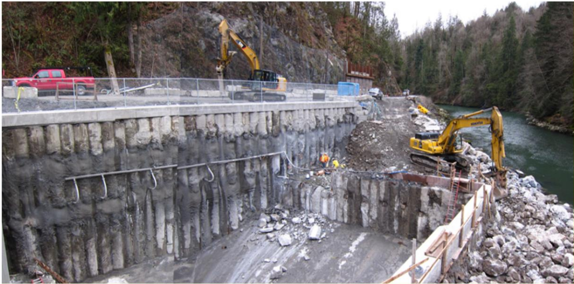
Figure 16-7: Typical Secant Pile Excavation Support
